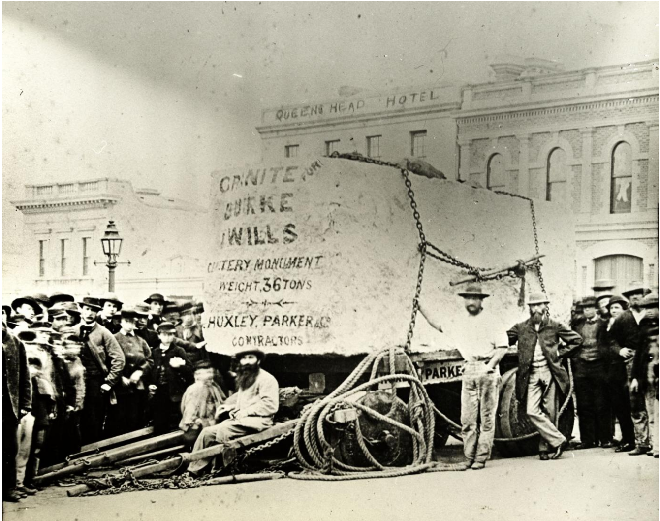
Figure 2 (State Library Vic) The large granite block parked in the centre of Queen Street. This appears from the newspaper reports to have been a planned overnight stop. The part not planned for was that the wagon sank into the road and it took all the next morning to jack and dig it out. Notice the front wheel has sunk about 9 inches into the road surface. The wheels were solid redgum slices with iron hoops around them. The load per wheel would have been about 7.5 tonnes so perhaps it is not surprising that some damage was done to the unsealed road surface. The well bearded man in the pale suit sitting on the shafts appeared in Figure 1. Was he Huxley or Parker or one of their employees?
