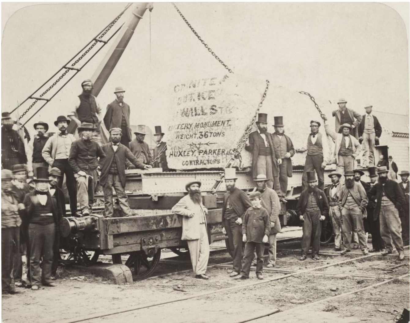
Figure 1 (State Library Vic.) The large granite block on arrival at Spencer Street Station in Melbourne. Note the stone is supported on a riveted iron frame suspended between two K class centre bolster flat wagons. The wagons are two of fifty built in 1859 by Joseph Wright and Sons in England, numbered 1K to 49K. They were designed to carry 8 tons each. The modification, which appears to be temporary, removed the springs and axle boxes and replaced them with rigid plain bearings. This lowered the height so the outer buffers were raised on offset packing blocks to lift them to the standard height. It seems that the stone on its supporting frame would have been within the standard Victorian Railways loading gauge, even without the reduction in height, so the lower bearings must have been to increase the load carrying capacity. Even so this load required a special train and was restricted to nine miles per hour with continual lubrication of the bearings. The crane visible in this photo is probably a pedestal crane rather than a mobile rail crane.
