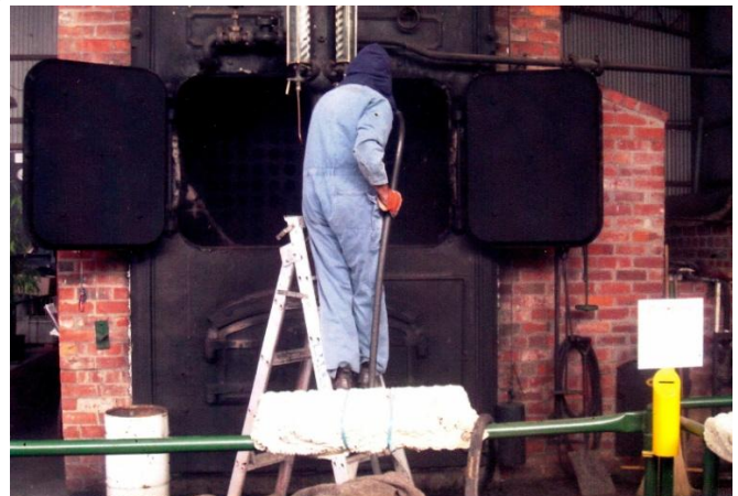
Leigh Buckley cleans the boiler with the air lance. The 94 3"φ tubes are 15' long
