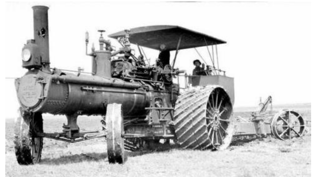
These American Traction Engines were used to direct ploughing the hard Prairie soil.
