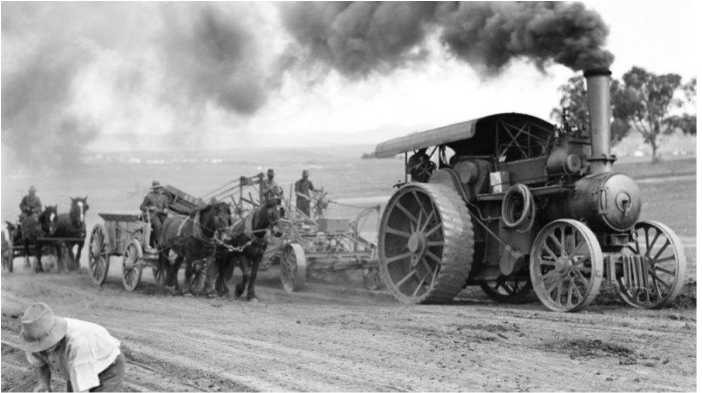
This Fowler Traction Engine was hard at work in 1925 forming the Roads in Canberra pulling a self elevating grader to fill horse drawn wagons. Still just 2 cylinders but it appears to be a compound.
