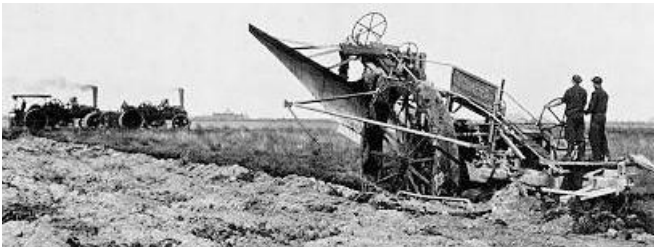
In the softer ground of Britain and Europe indirect ploughing was done by a cable between two ploughing Engines. About 100 of these engines are thought to have come to Australia. The Scienceworks Fowler Ploughing engine will be at the rally in May.
